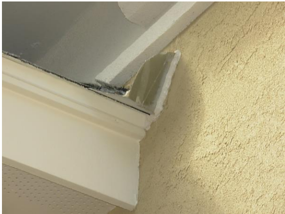
Kick out flashing at roof/wall intersections
