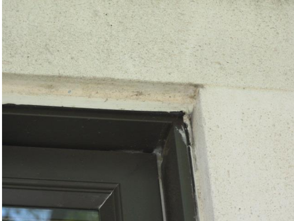
Metal head flashing at top of windows
